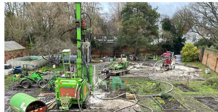
GSHP ground array installation at Bell House, Dulwich.
