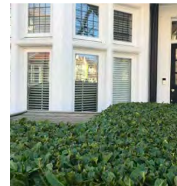
Leaded glass can have internally fitted secondary glazing
