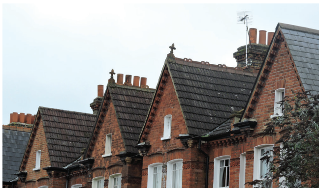
Post war concrete tiles should be replaced with original tiles
