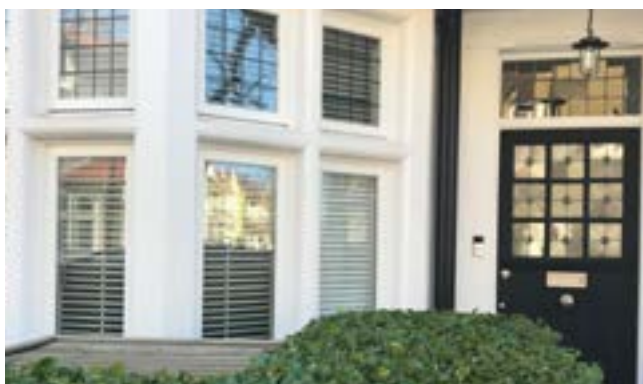
Like-for-like window replacement
