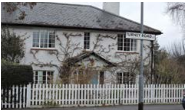
Original steel window replacement
