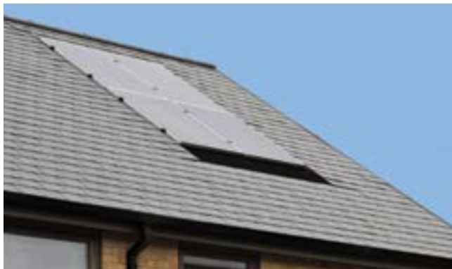
In-line solar panels
