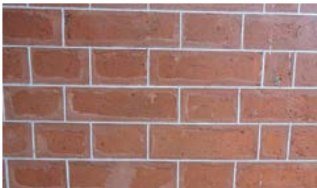
Suitable tuck pointing
