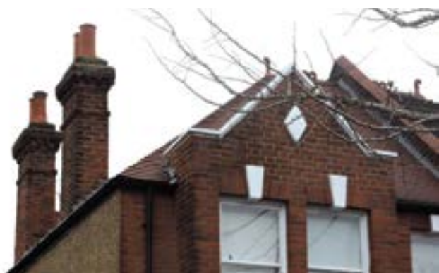
Chimney stack Desenfans Road
