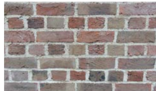
Suitable flush pointing
